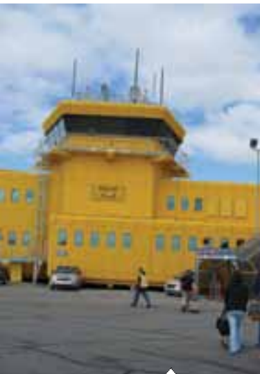
Iqaluit Airport Terminal Building SOURCE: CBC.ca
