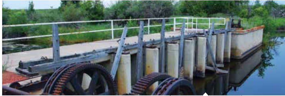
Magrath Canal Headworks SOURCE: Alberta Culture 2008
