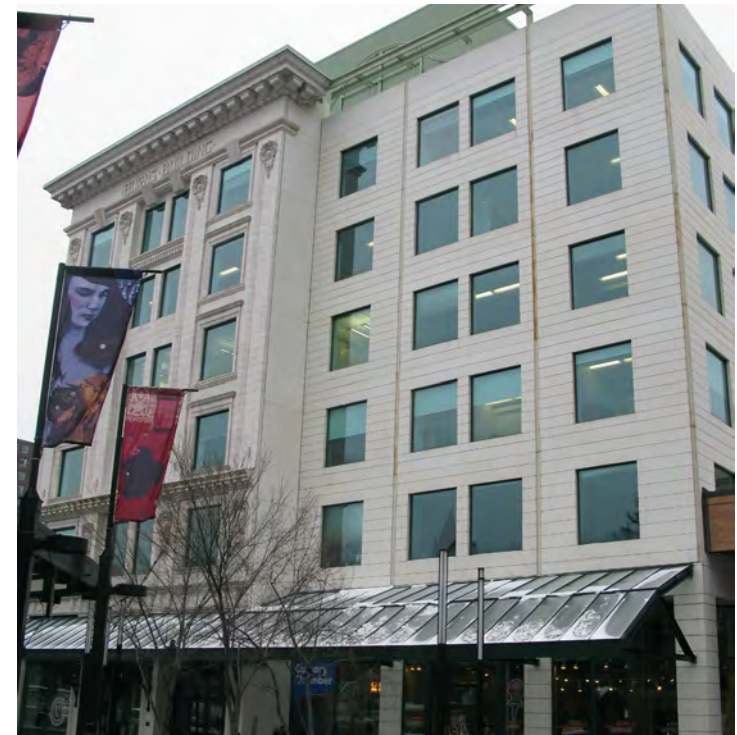
This contemporary development is respectful of the adjacent heritage building to its left, using compatible fenestration (or window treatment), cornice lines, awnings and cladding materials.
