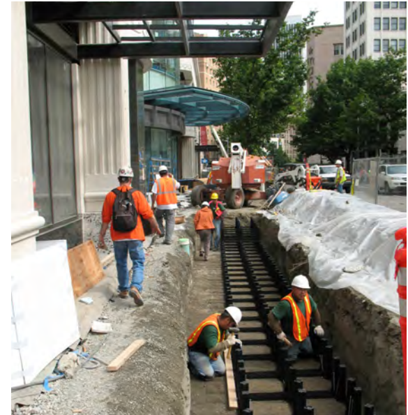
This modular structure for tree boulevards should prevent damage of adjacent pavement and underground utilities by spreading roots and will provide predictability for future nearby work under the pavement.
