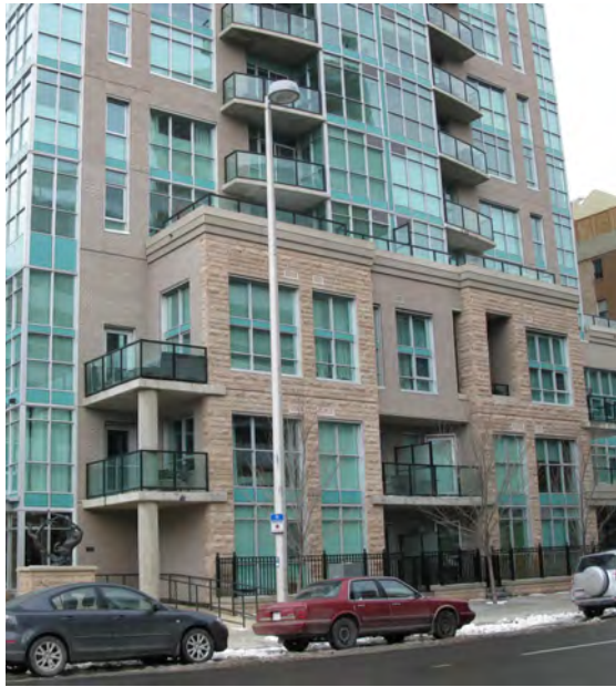
Residential podium (or base building).
