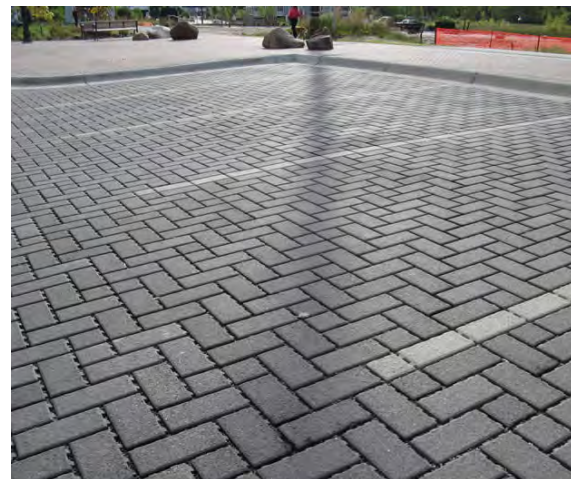
Permeable paving can be used to provide increased stormwater infiltration and minimize runoff.
