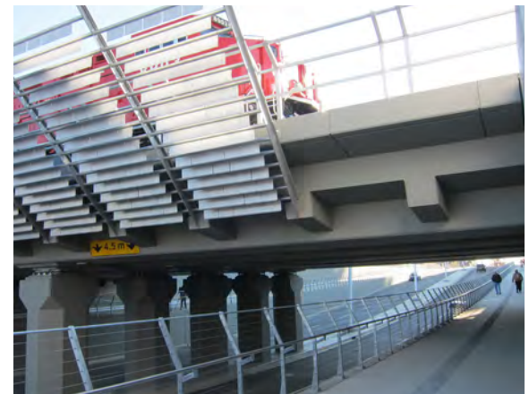
Off-street, multi-use pathway at 4 Street SE underpass.
