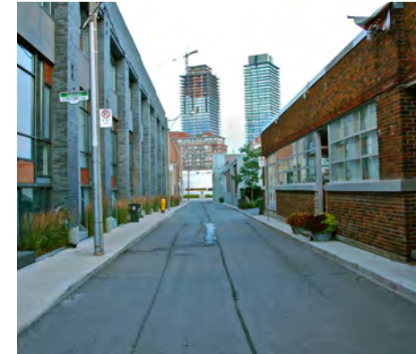
Service lanes with green edges and on-site bio-filtration planters contribute to sustainable stormwater management.
