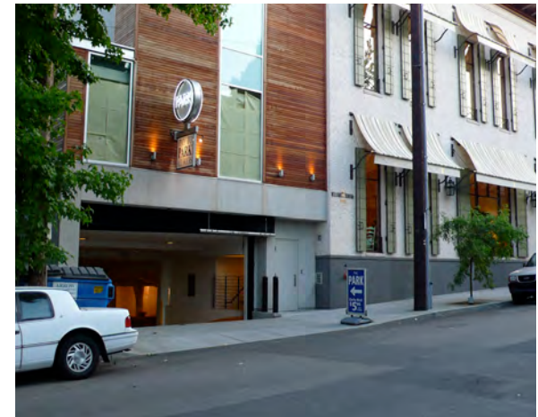
Limit the number and width of vehicle entries along a street frontage to maximize continuity of street wall and the public realm.
