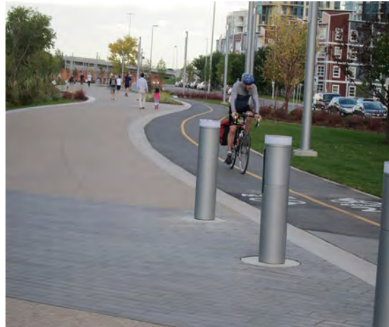
Varied paving materials at this multi-use pathway help to define pedestrian and cyclist zones and highlight potential conflict zones (i.e. pedestrian crossing).
