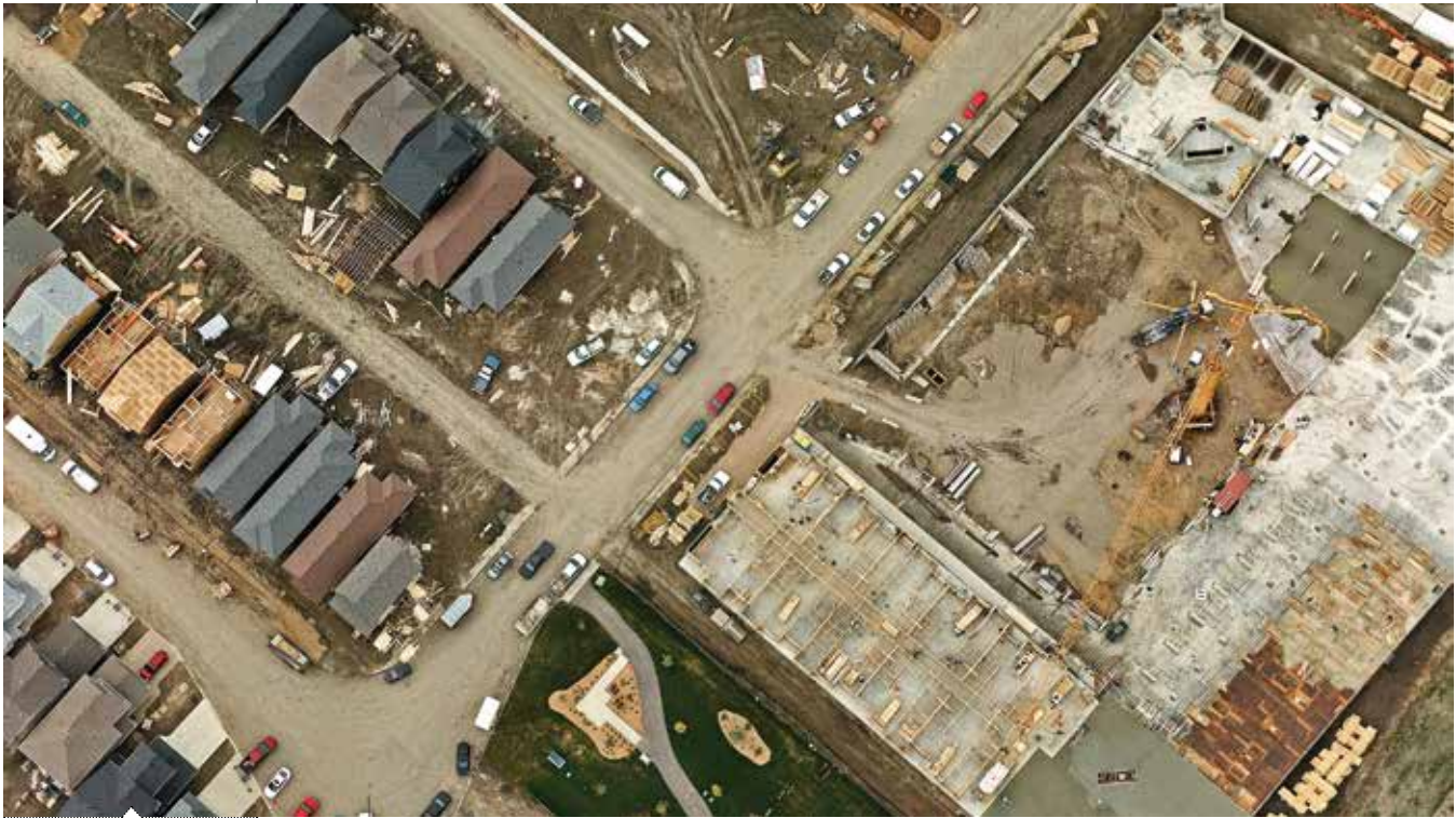
A development under construction, Regina, 2013.
