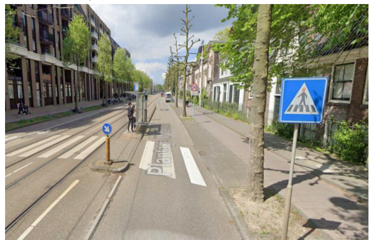
Google (2024). Four traffic calming mechanisms in one image. Placing tall trees close to traffic both protects cyclists from errant motorists and gives the impression of a narrower lane, as does the slight change in elevation between the traffic and tram lanes. The curve in the station platform forces drivers to slow down, counteracting the street's long stretches between intersections. Further ahead, we see a “Busvriendelijke drempel” or bus-friendly bump, a speed bump designed to slow cars while letting buses and emergency vehicles go unimpeded (Struyk Verwo Infra).
