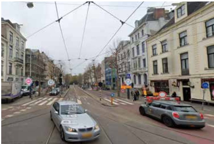
Google (2024). Plantage Middenlaan, facing west. Note the separated tram, car, and bike lanes (bike lanes closed due to COVID-19), and median pedestrian islands to make crossing the street more comfortable.
