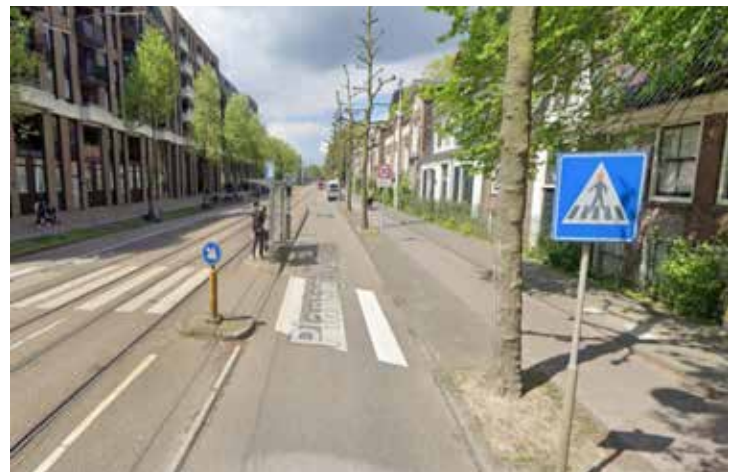
Google (2024). Four traffic calming mechanisms in one image. Placing tall trees close to traffic both protects cyclists from errant motorists and gives the impression of a narrower lane, as does the slight change in elevation between the traffic and tram lanes. The curve in the station platform forces drivers to slow down, counteracting the street's long stretches between intersections. Further ahead, we see a “Busvriendelijke drempel” or bus-friendly bump, a speed bump designed to slow cars while letting buses and emergency vehicles go unimpeded (Struyk Verwo Infra).
